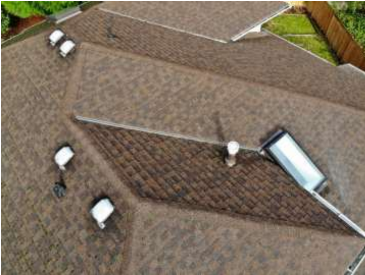
Roof, high ridge
