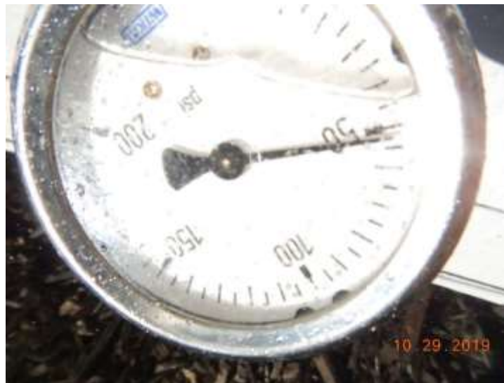
Water pressure is adequate and not excessive
