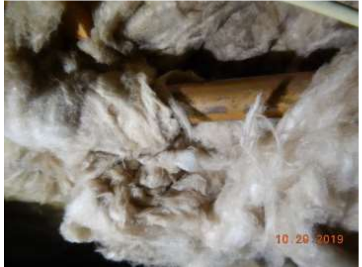
Domestic water distribution pipes
